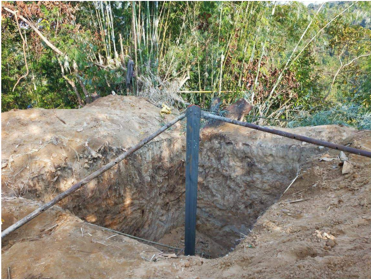
Figure 2.5 Photograph setting template being prepared for final concreting
