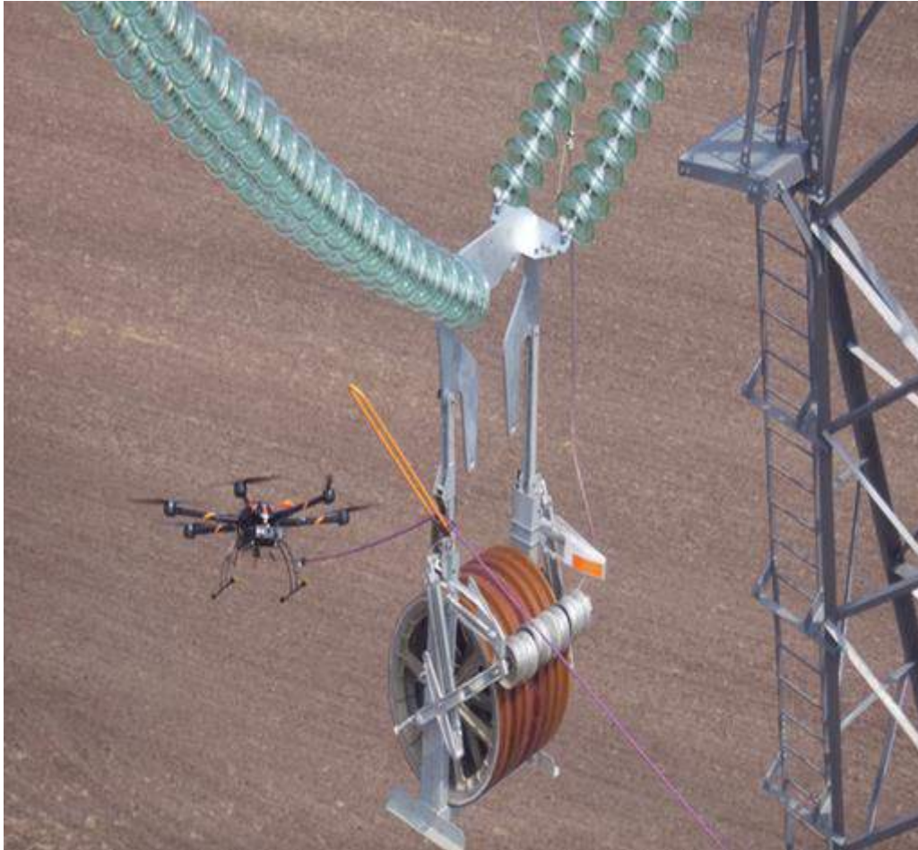
Figure 2.7 Conductor Stringing
