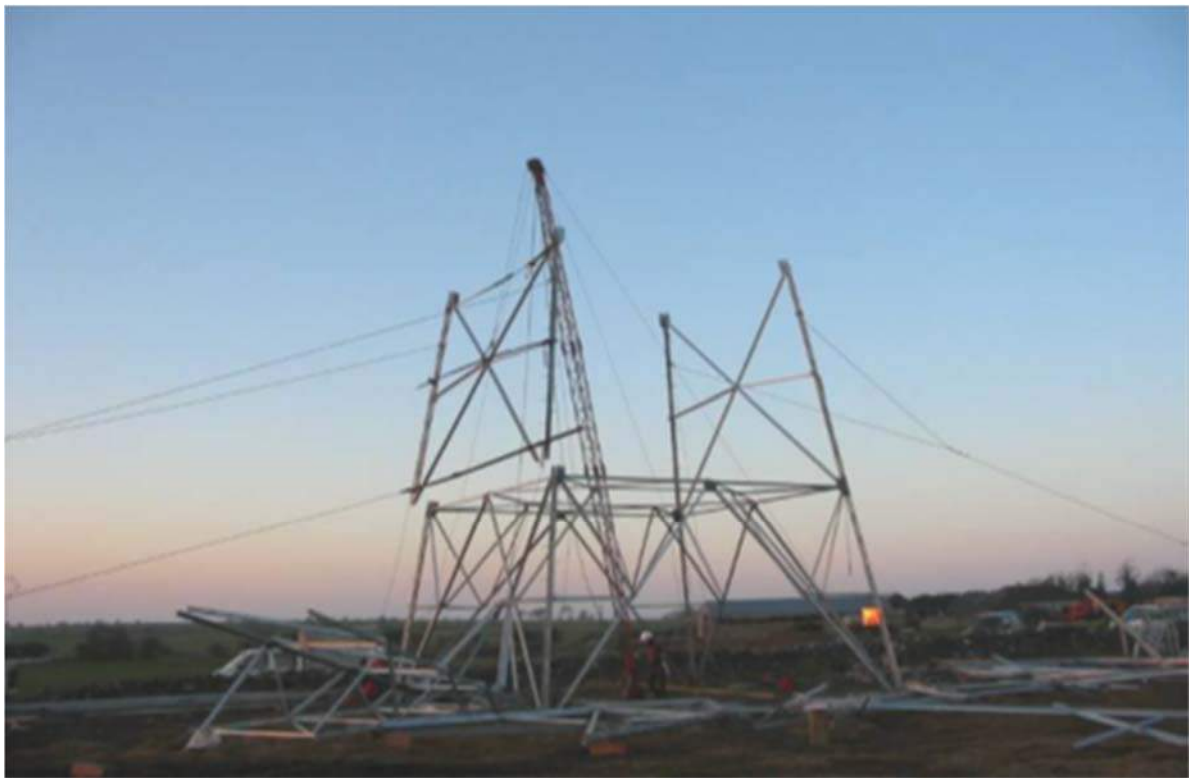
Figure 2.4 Model visual: Derrick pole at tower base
